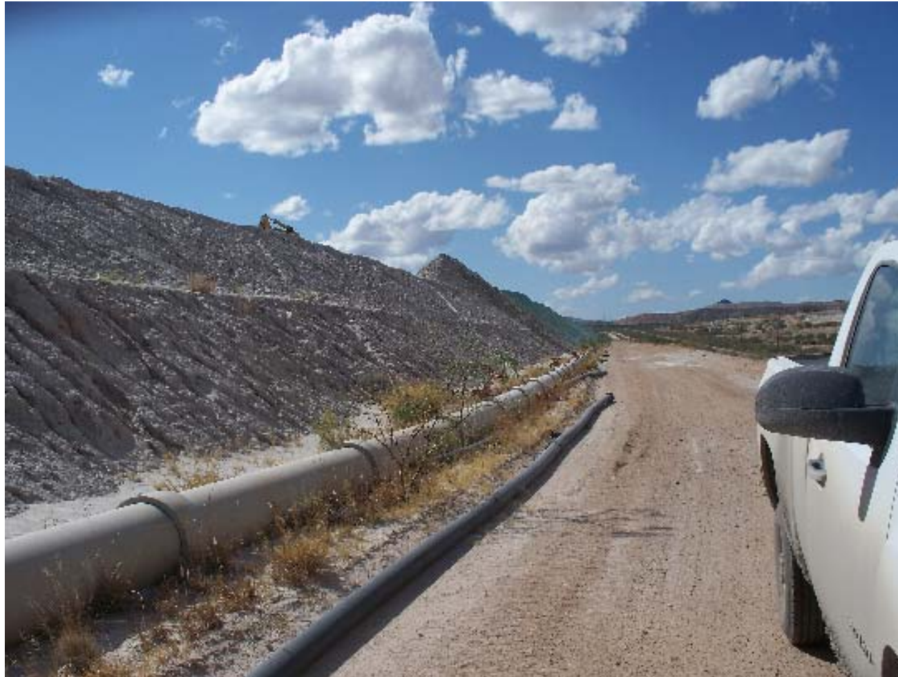
Berm Building Area. North side of Tailing # 8. Berm building stopped
